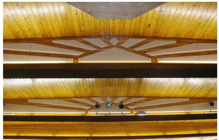
Ceiling beams with acoustics, facing speaker
